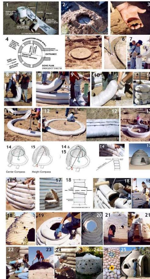
Figure 2 The building process of Superadobe
